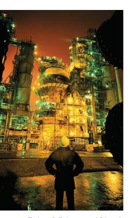
The large distillation tower at left is used to separate petroleum into fractions based on their boiling points. The "cat cracker" at right uses catalysts and high temperatures to crack large molecules into smaller ones.
