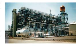
This plant in Tokuyama, Japan, passes ethane rapidly over a hot catalyst. The products are ethylene and hydrogen.
