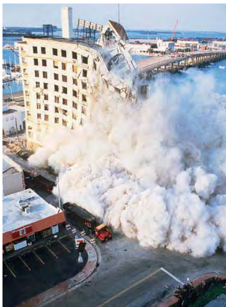
FIGURE 20.4 Chemical explosives are used to demolish a building in Miami, Florida.
