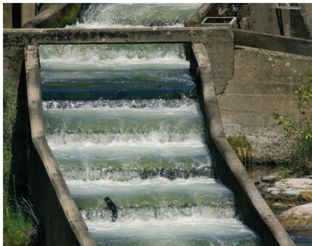
FIGURE 27.3 Fish ladder. Because dams are an impediment to fish such as salmon that migrate upstream to breed, fish ladders like this one on the Rogue River in Oregon have been designed to allow the fish to get around the dam and continue on their traditional path of migration. (Kevin Schafer/Alamy)
