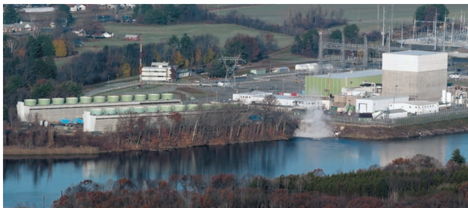
FIGURE 44.3 Thermal pollution. Nuclear reactors, such as the Vermont Yankee nuclear plant, use water to generate steam. To cool this steam, they either use cooling towers or empty the water into holding ponds. In both cases, the water must be cooled before it is returned to the natural source of water such as a lake or river. In 2013 the owners of Vermont Yankee announced they would not seek to renew their license. (CJ Gunther/epa/Corbis)
