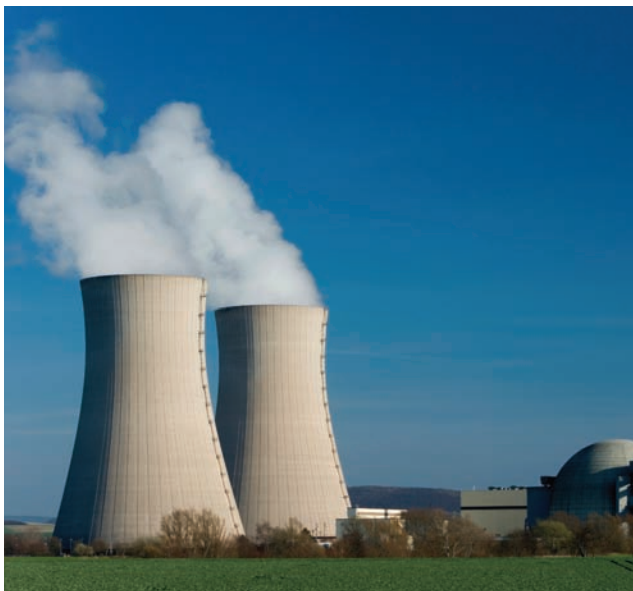
FIGURE 28.4 Water consumption in nuclear power plants. When nuclear reactors, such as this one in Germany, heat water to make the steam that turns electrical turbines, the steam must be cooled back down. During the cooling of the steam, a great deal of water vapor is released to the atmosphere. (Hans F. Meier/iStockphoto.com)
