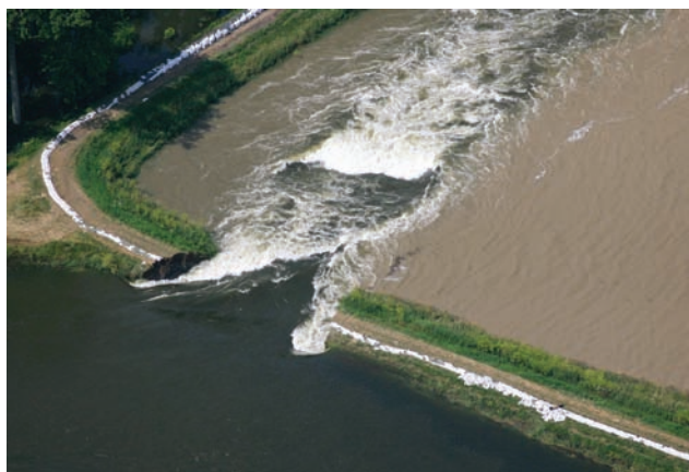
FIGURE 27.1 Levees. Levees are built to prevent rivers from flowing over their banks and onto the floodplain. In 2008, this levee, just north of St. Louis, Missouri, collapsed and allowed the floodwaters to spread over the surrounding fields. (Anthony Souffle/MCT/Landov)
