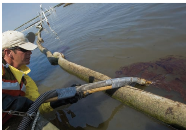
FIGURE 43.3 Oil-spill containment. Floating plastic walls can contain oil spills while the oil is sucked off the surface of the water. (Matthew Hinton/The Times-Picayune/Landov)
