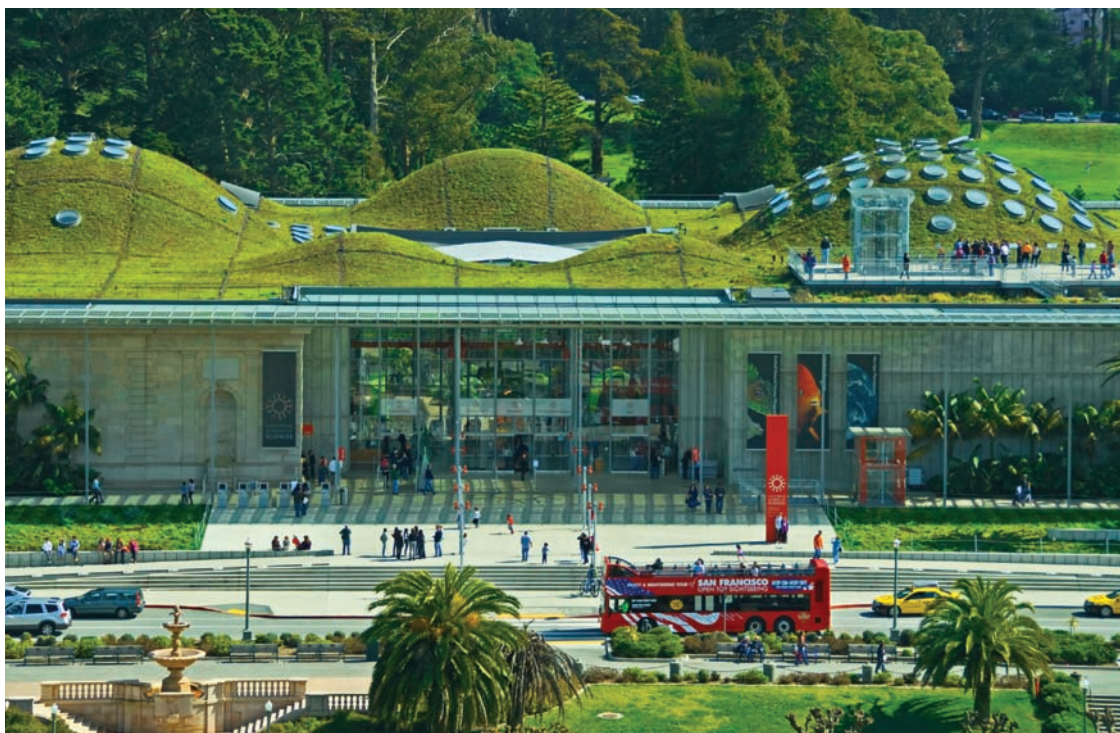
FIGURE 37.4 The California Academy of Sciences. The sustainable design of this San Francisco research institution maximizes the use of natural light and ventilation. The building generates much of its own electricity with solar panels on its roof and captures water in its rooftop garden. (Nancy Hoyt Belcher/Alamy)
