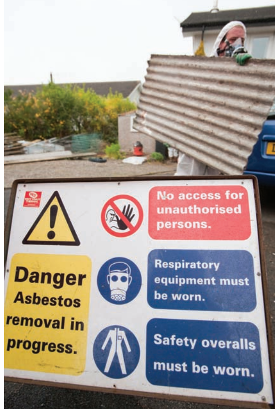
FIGURE 58.5 The risks of asbestos dust. Despite nearly a century of studies on the risks of asbestos dust to human health, only recently have workers been required to go to great lengths to prevent exposure. Today, they dress in chemical suits and respirators when removing asbestos from a building. Applying the precautionary principle would have required protection of workers many decades earlier and saved hundreds of thousands of lives. (Ashley Cooper/Alamy)
