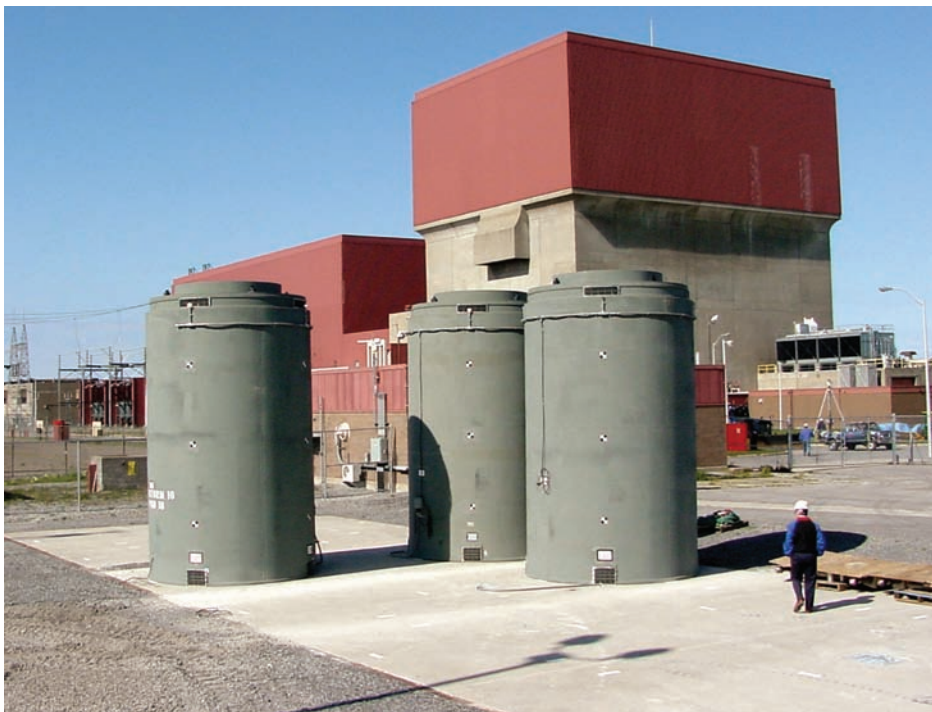
FIGURE 36.3 Storage of nuclear waste. Nuclear waste is often stored in metal containers at the power plant where it was produced. (AP Photo/Holtec International)
