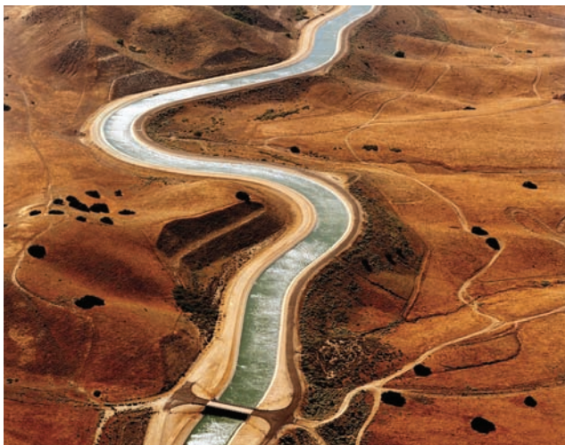
FIGURE 27.4 Aqueducts. Aqueducts deliver water from places where it is abundant to places where it is needed. This section of the Colorado River Aqueduct, which diverts water from the Colorado River to Los Angeles, passes through the Mojave Desert. (Mark Hanauer/Corbis)
