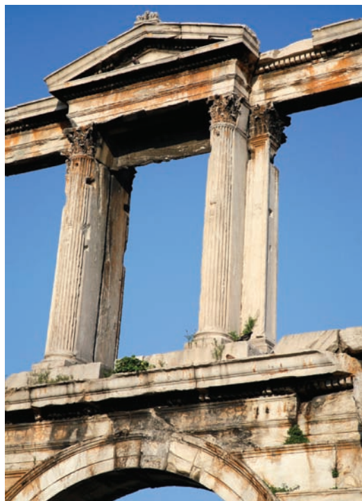
FIGURE 47.4 Material damage from acid deposition. Hadrian's Arch, near the Acropolis in Athens, Greece, has been damaged by acid deposition. It is made of marble, which contains calcium carbonate, and is susceptible to deterioration from acid deposition and acids in the air. (Sites & Photos/HIP/The Image Works)
